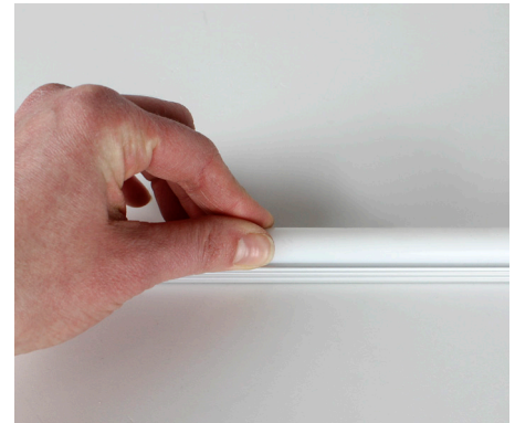
Installing the Light
